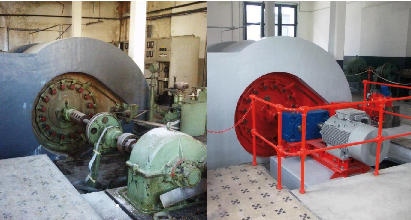
Turbine Francis Bergamo
